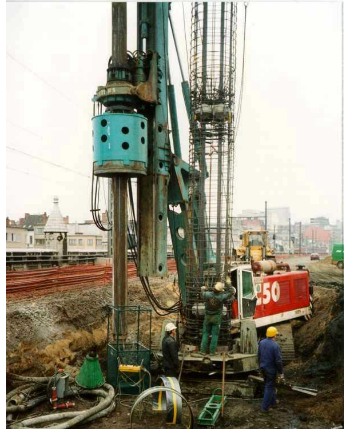
Figure 4b: Installation of the reinforcement cage
