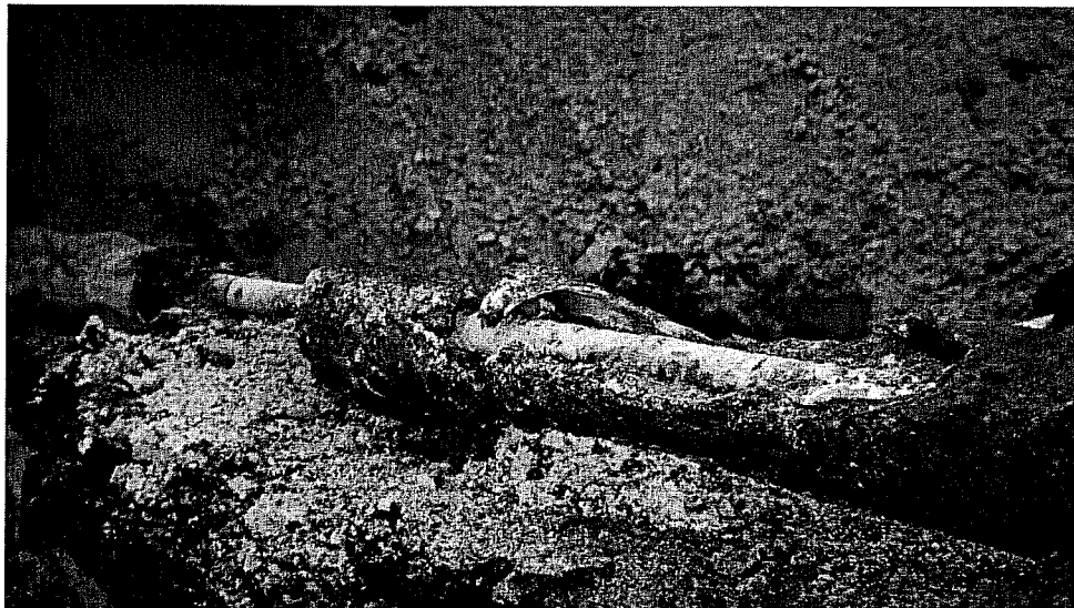
Figuur 8h: Holte in cementomhulling
