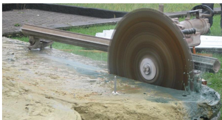
Figure 4: Sawing of a CSM panel
