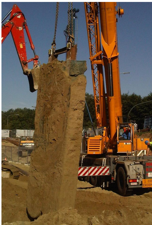
Figure 3: Excavation of an in situ executed CSM panel (Lameire Funderingstechnieken n. v.)
