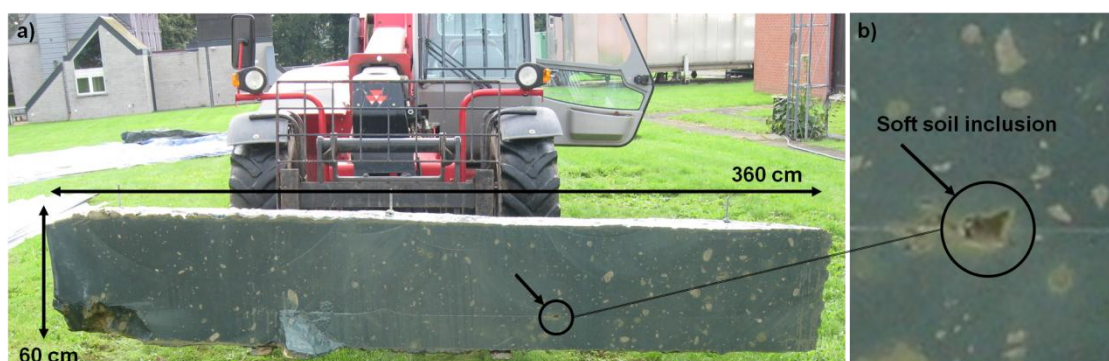
Figure 2: a) Saw-cut section of a CSM panel, b) enlargement of a soft soil inclusion
